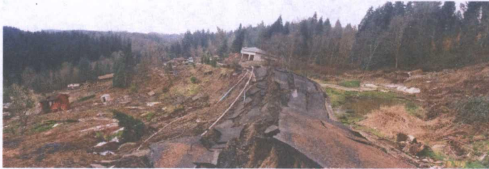
Photo of landslide damage, Photo from Dr. J David Rogers
